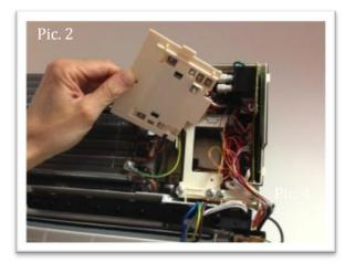
3) Insert the CAB-SERV cable from the rear of the indoor unit into the trough-hole toward the front side, just near the indoor unit PC Board (pic. 3, 4).
