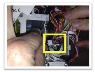
5) Connect the ground wire of CAB-SERV on a ground tab available on the indoor unit.
